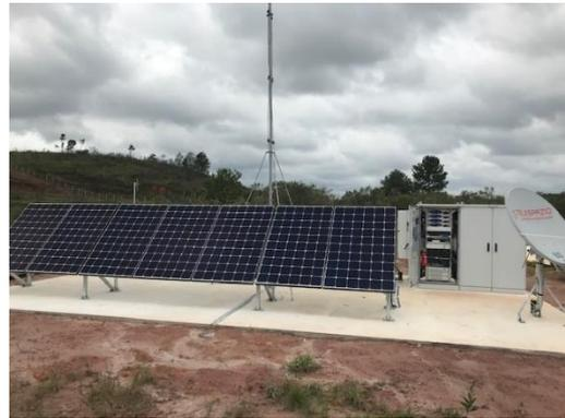
Everything else could be supplied as an integrated system with minimal ground works, outdoor cabinets, masts and sensors.
